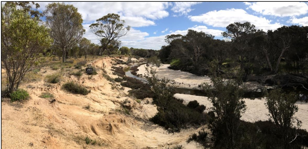
Figure 8: Typical features of the main channel of Warperup Creek are a relatively narrow floodway.
